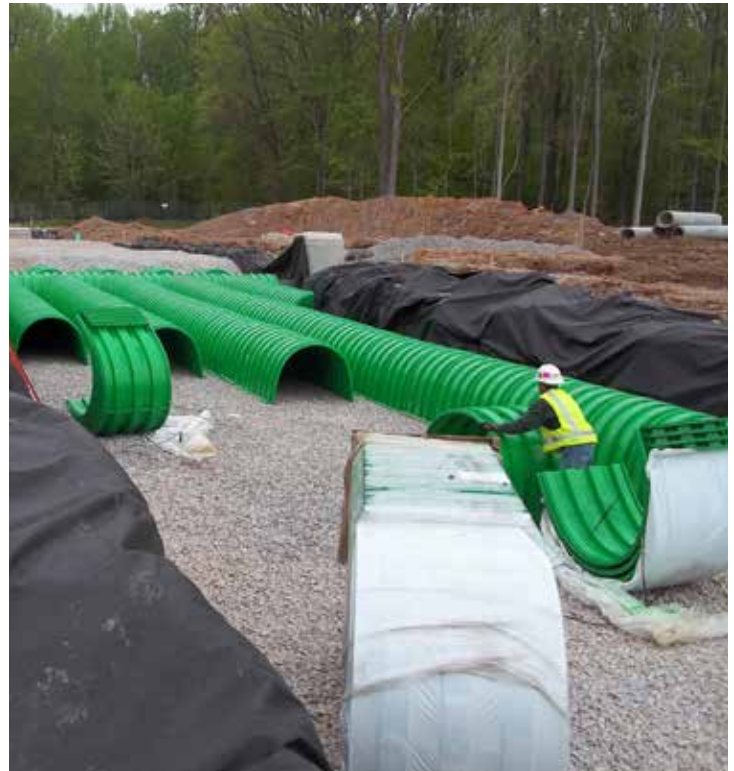
Infiltration basin immediately after a storm event (Left). Installation of subsurface detention cell (Right). Photo Credits: ACT Engineering, Inc.
